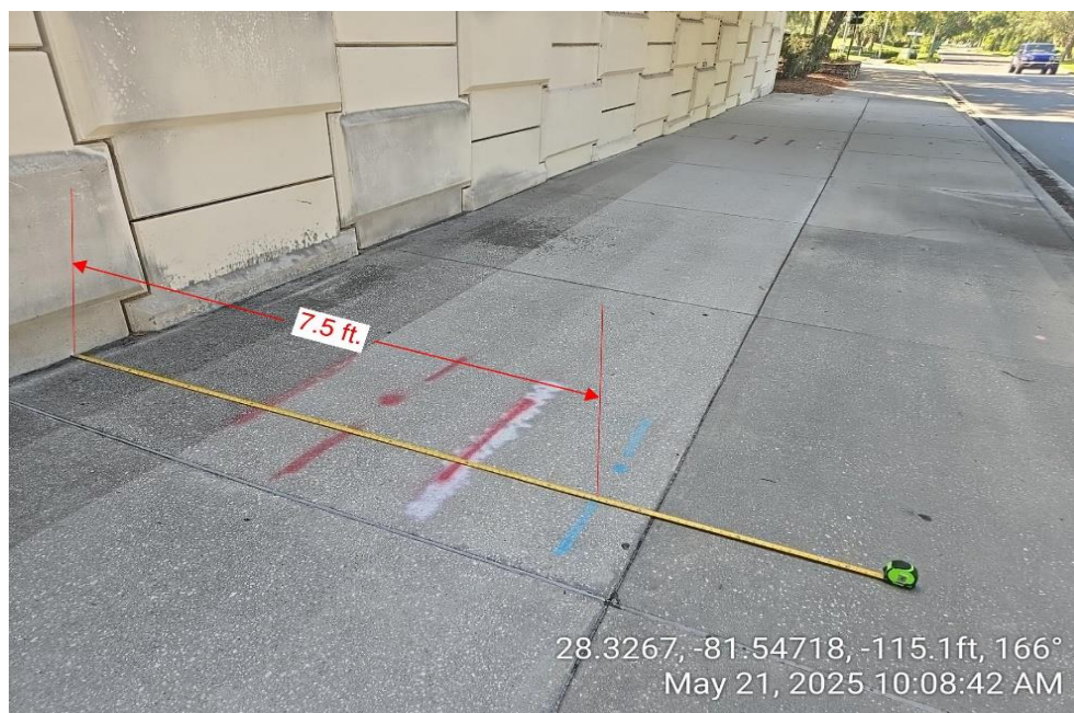
Underground 16-inch diameter water main is 7.5 feet away from proposed piling activity at the MSE wall.
